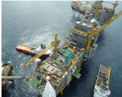
Johan Sverdrup Riser Platform hook-up and modification
