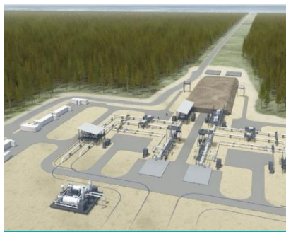
Nord Stream 2 onshore facility
